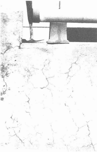
FIGURE 3: Bridge Structure constructed in 1980. Moderate reaction after 4 years.
