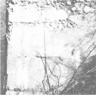
FIGURE 8 NO MAP-CRACKS 78 YEAR OLD CONCRETE
