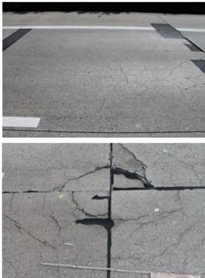
Figure 1.1: Examples of the deteriorated areas of pavement from the expressway
