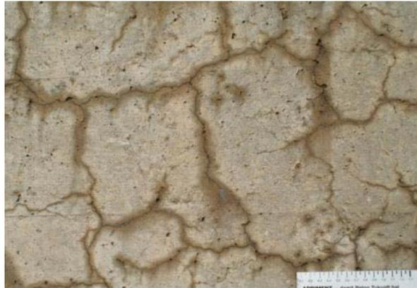
Figure 1.1: Typical crack pattern caused by ASR. Horizontal field width = 50 cm.
