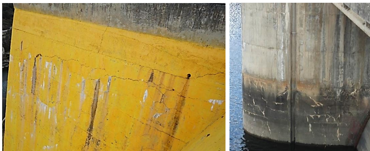
Figure 1.4: Map cracking at the top of the left abutment (left image) and on the right surface of pier 1D, upstream (right image) (photos taken in June 2019)
