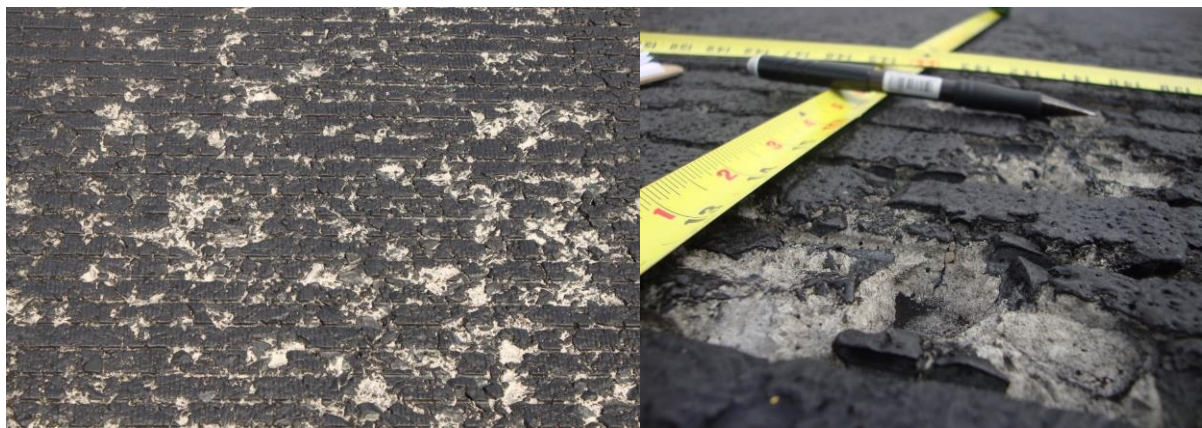
Figure 2.1: Examples surface distress (popouts and loss of paste).
