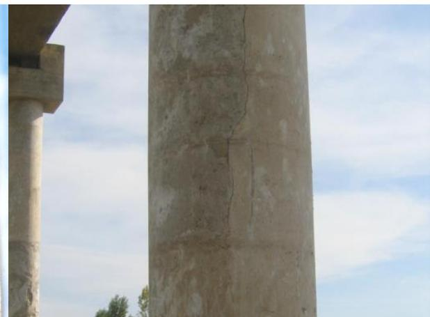
Figure 4.2: Cracking in pillar of Channel E
