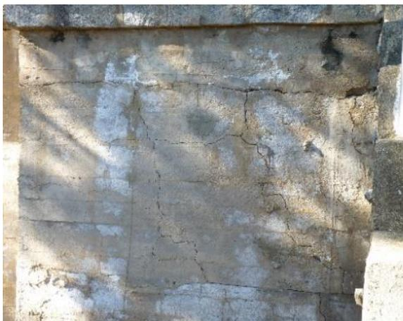
Figure 4.1: Cracking in DAM C
