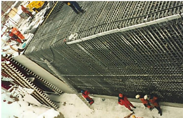
Figure 1.1: Outer wall and top slab during construction of the Maridal culvert in Oslo, Norway [1].
