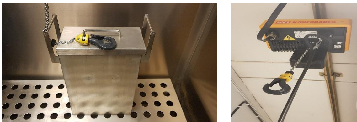
Figure 3.3: Example of suitable health and safety measures for easy handling of the containers.
