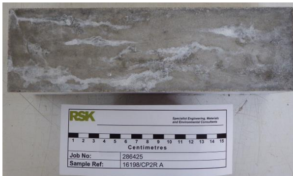
Figure 2.6: White deposits on the surface of concrete prism (Mix 2)
