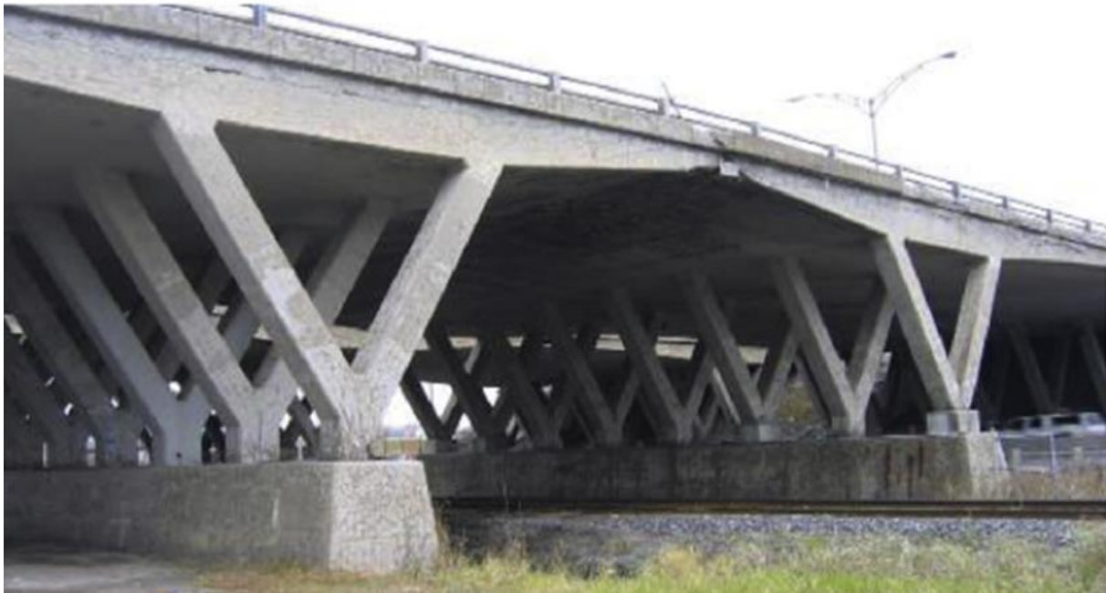
Figure 4.1: RBC overpass after nearly 50 years in service [15].
